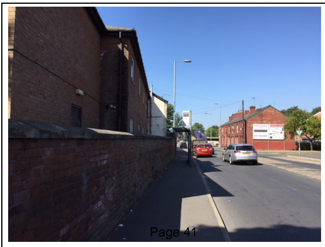
Photo 6 - view looking westwards along northern boundary of the site with Oxford Road
