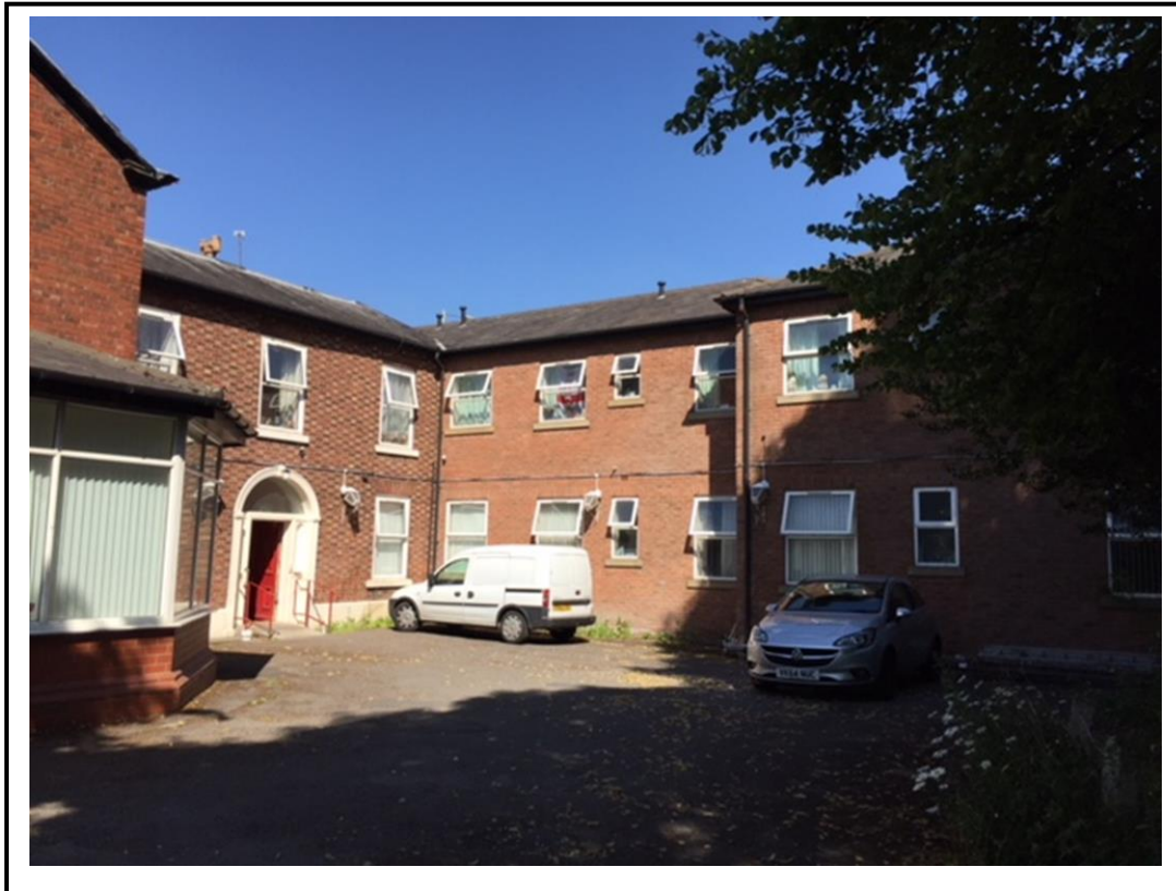
Photo 5 – view of car parking area to the front of the building
